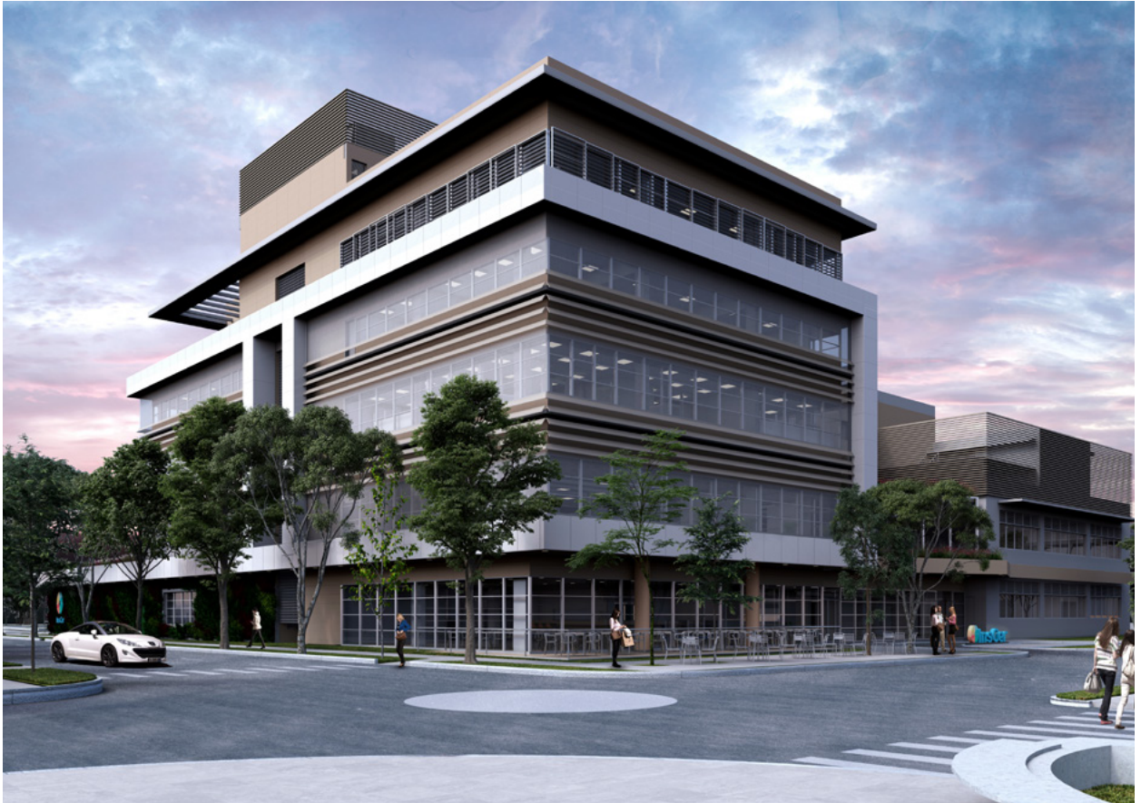
New building will be three times as large and will be ready in 2020
